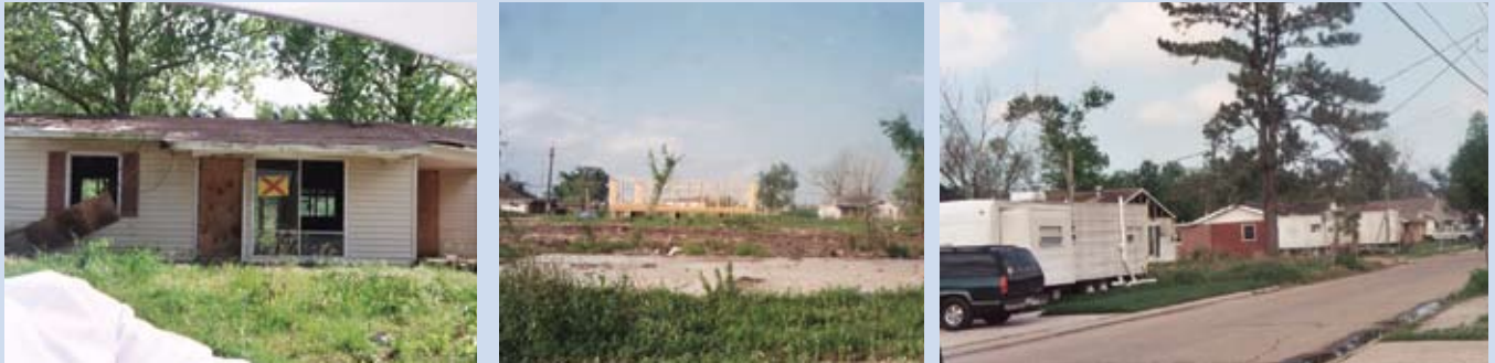
Reality in a New Orleans parish (from left to right)—A home marked for demolition with the unmistakable FEMA “X”; empty foundations where homes once stood, with some scattered signs of rebuilding; “temporary” FEMA trailers that have become homes for residents trying to rebuild.
