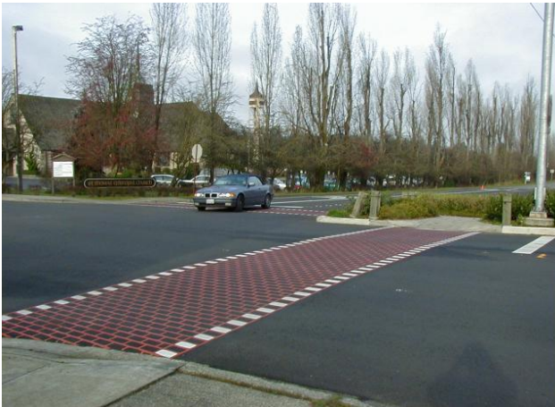
Bricking can make the crosswalk more visible and the neighborhood more distinctive
